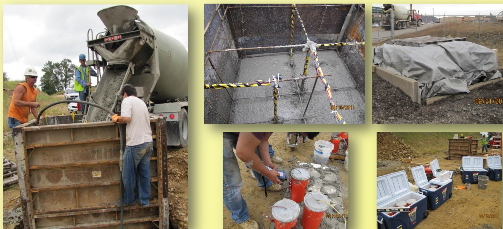
Figure 2- Cube construction, concrete pouring, placement and making concrete cylinders.
